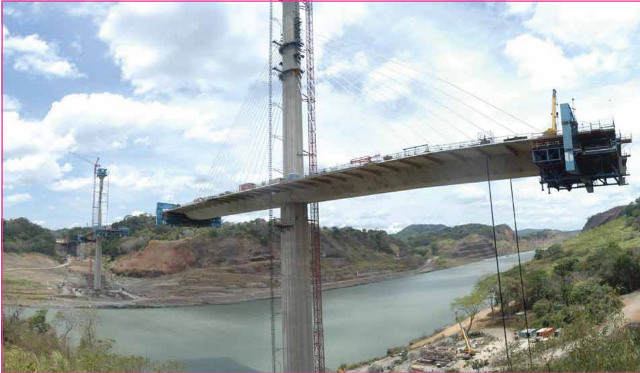
Construction of the "Second Bridge over the Panama Canal - Republic of Panama" for which EURO PRESS has supplied the hydraulic components that hold the segments for the construction of the floor system of the bridge (Panama, July 2003)
